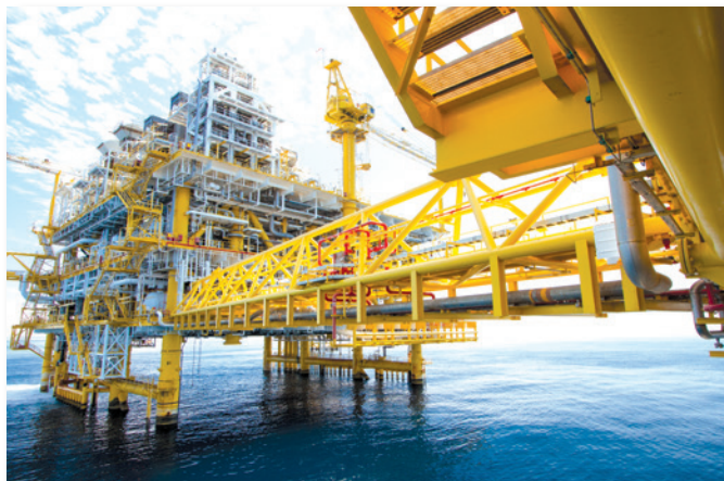
Operating platform in deep water up to 520m, anchored by concrete legs to the ocean floor.
